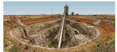
Incline conveyor and silo at Zibulo Mine in RSA. AnnRpt 2011, p67.
